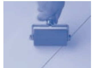
Step 4 Roll edges, seams, field of roof
