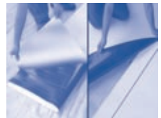
Step 3 Remove release film (left) and adhere membrane (right)
